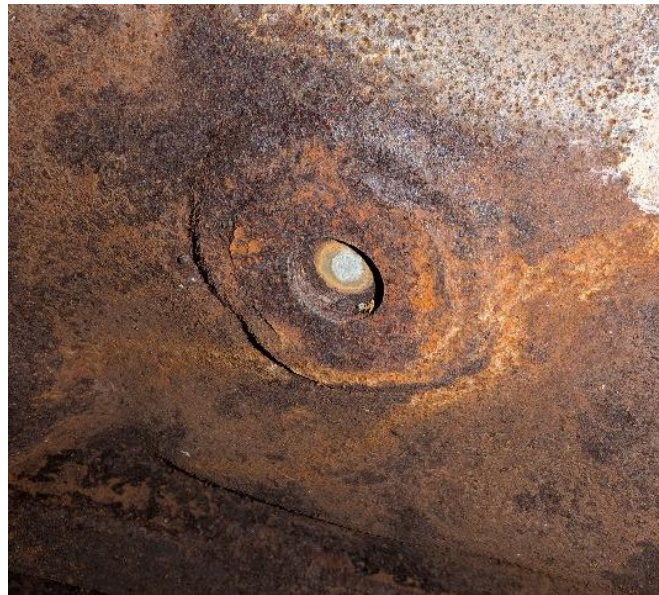
FIGURE 6: THE FUSIBLE PLUG AS SEEN FROM THE INSIDE OF THE CYLINDER HEAD, WITH ITS DISTINCTIVE BIMETALLIC CONSTRUCTION VISIBLE
