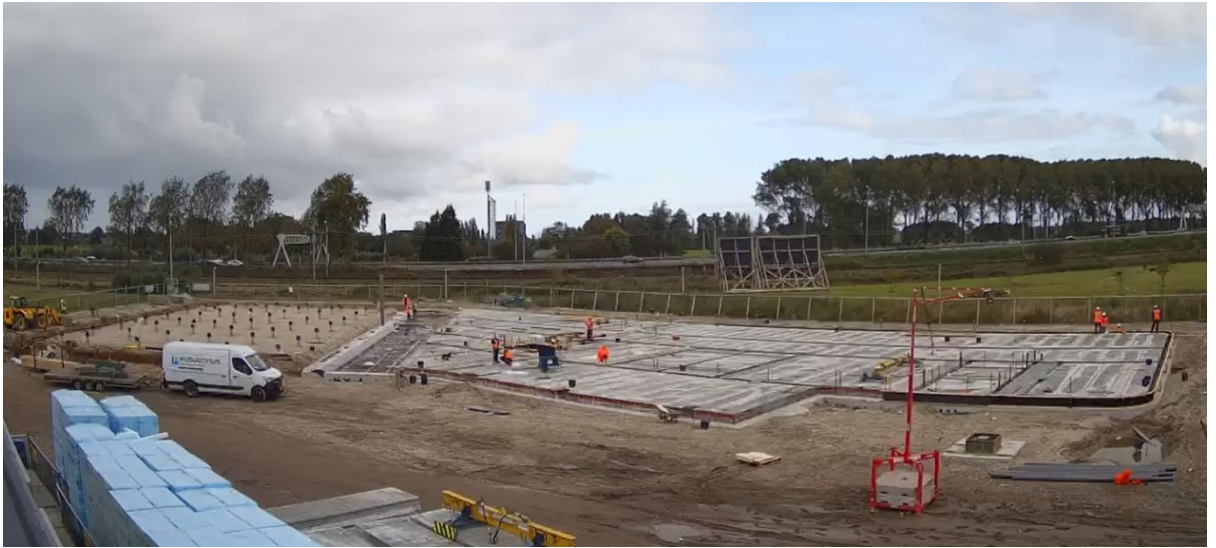
FIGURE 2: PLACEMENT OF THE PREFABRICATED GROUND FLOOR (11 OCTOBER 2021)
