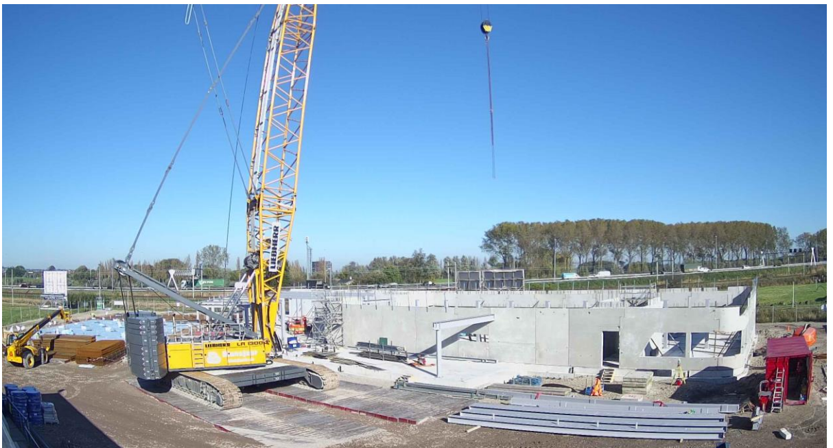
FIGURE 3: MOUNTING OF THE PREFABRICATED CONCRETE STRUCTURE (28 OCTOBER 2021)
