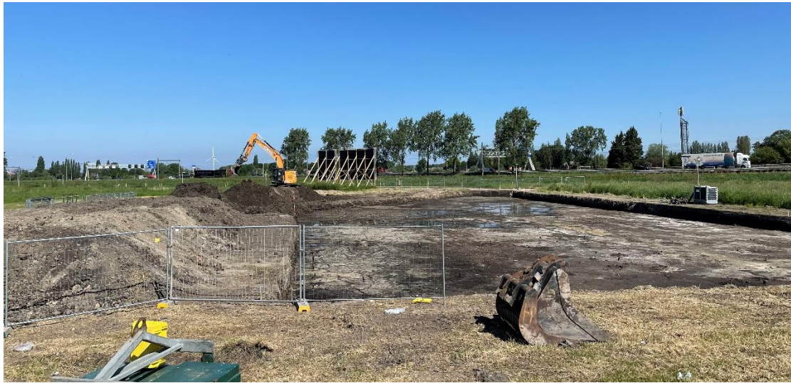
FIGURE 1: START OF THE FIRST GROUND WORK ON SITE (10 JUNE 2021)
