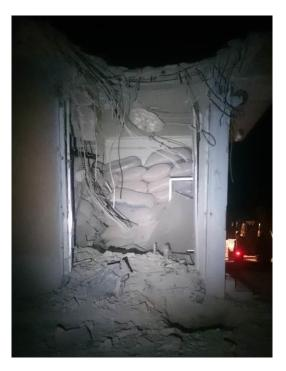
6.30 Figure 12 is a photograph taken on the morning after the day of the reported incident. The damage can be observed from a different angle. The position and shape of the metal rebar protruding from the reinforced concrete indicates that the damage was caused by a force exerted from above.
